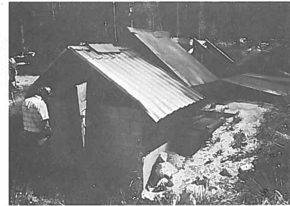
(a) Effluent end of filter outside the valve meter area.
