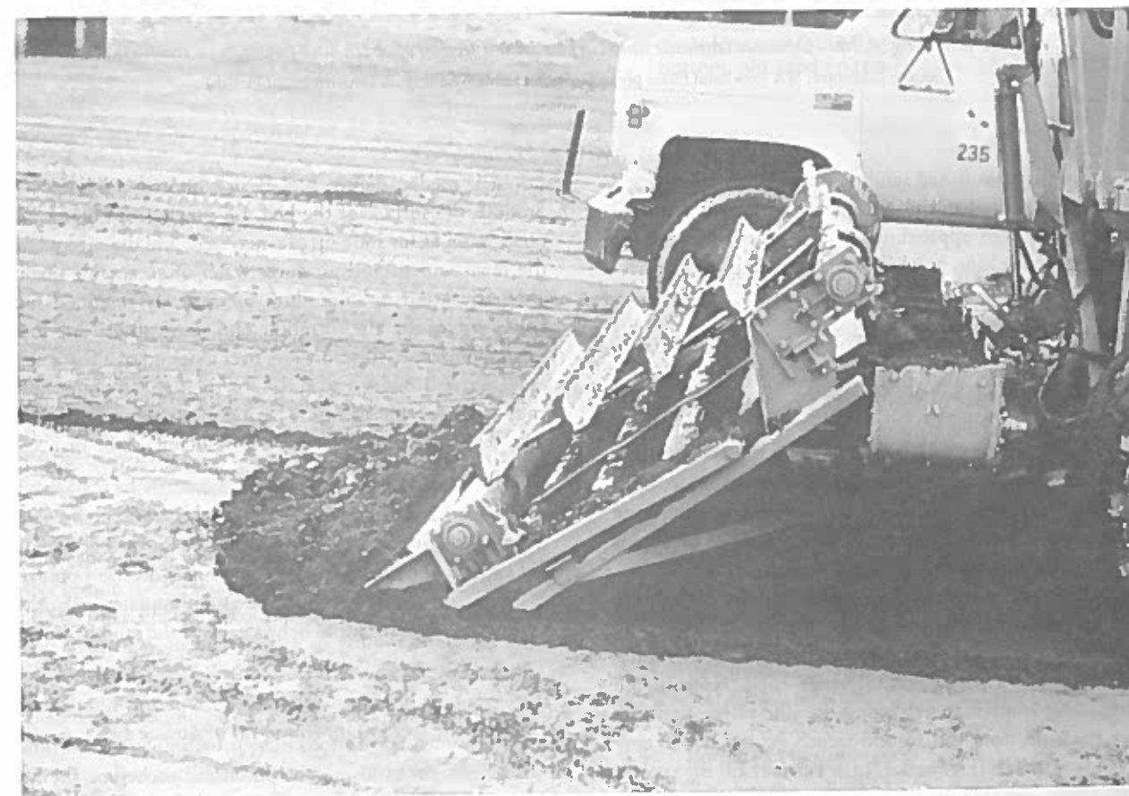
Fig. 4.25 Mechanical equipment used for cleaning a large slow sand filter (Source: Salem, OR Water/Wastewater District)
